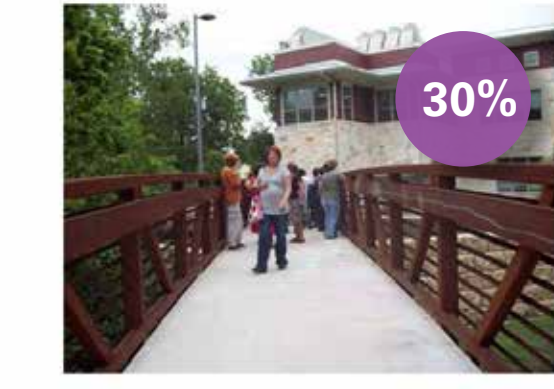
3. Bridge Over Creek
